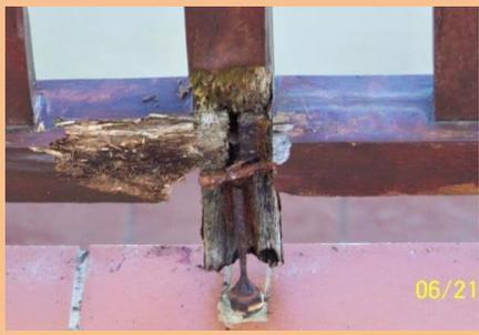
The balustrades are likewise about 20 years old too and some need to be replaced as a matter of urgency as some are currently unsafe due to the wood rotting – as can be seen from the photo on the left. Research has indicated that there is a severe lack of providers for the current product and after consultation with our architect on the right product to use, it has been agreed to change to stainless steel balustrades (SABS approved, a product that can sustain the seaside climate).
