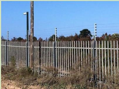
Electric Fence: The entire perimeter fence was risk assessed and found to be deficient in several areas. Due to the Estates proximity to the lagoon the original electrification of the fence over the last twelve years had deteriorated to the extent that it could no longer carry the required voltage at all times.
